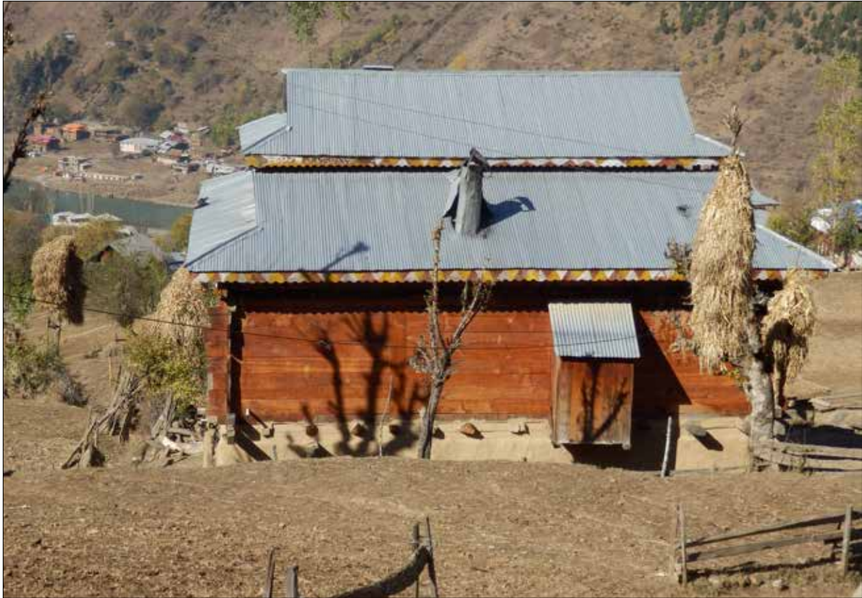
Figure 8. Chimney to emit smoke and suspended washroom (Photograph: Authors).
