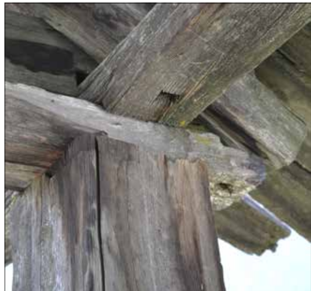
Figure 18. A specimen of Dovetail joint or Chul system (Photograph: Authors)
