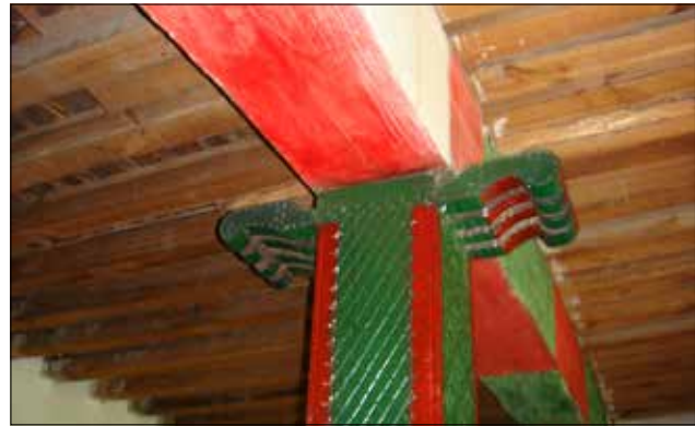
Figure 17. Central vertical post and beam (Photograph: Authors)
