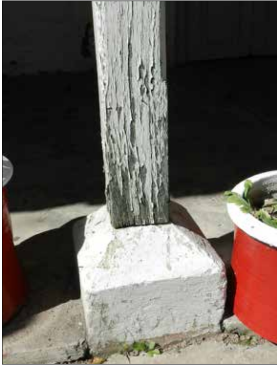
Figure 3. Stone-base of wooden post to be fixed in ground (Photograph: Authors).
