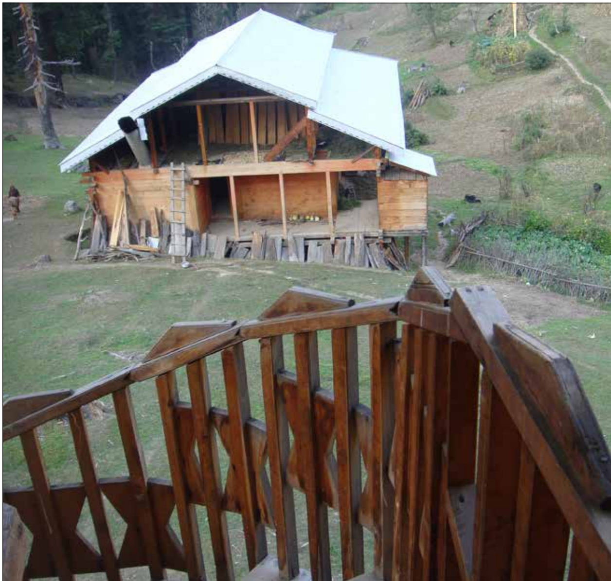
Figure 27. Modern wooden house under construction and winding staircase (Photograph: Authors)
