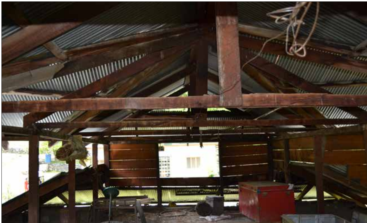
Figure 15. Interior of attic with pronounced cross ventilation (Photograph: Authors).
