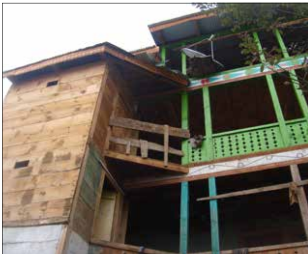
Figure 25. Perforated grills and decorative eaves (Photograph: Authors)
