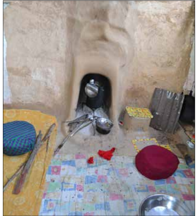
Figure 10. Fire place with mud-plaster coating (Photograph: Authors).
