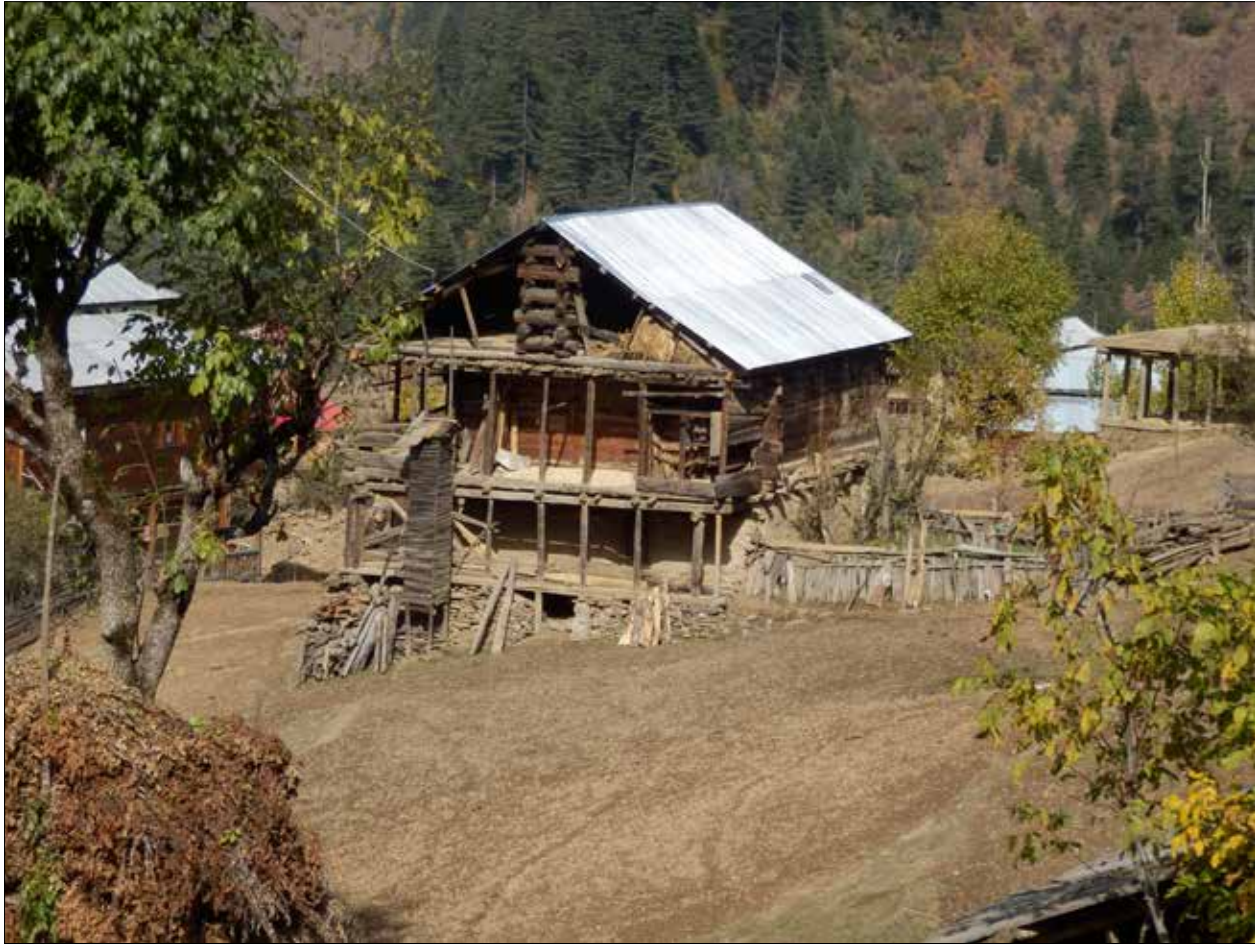
Figure 2. An old house (may be more than hundred years of age) in Shāradā (Photograph: Authors).
