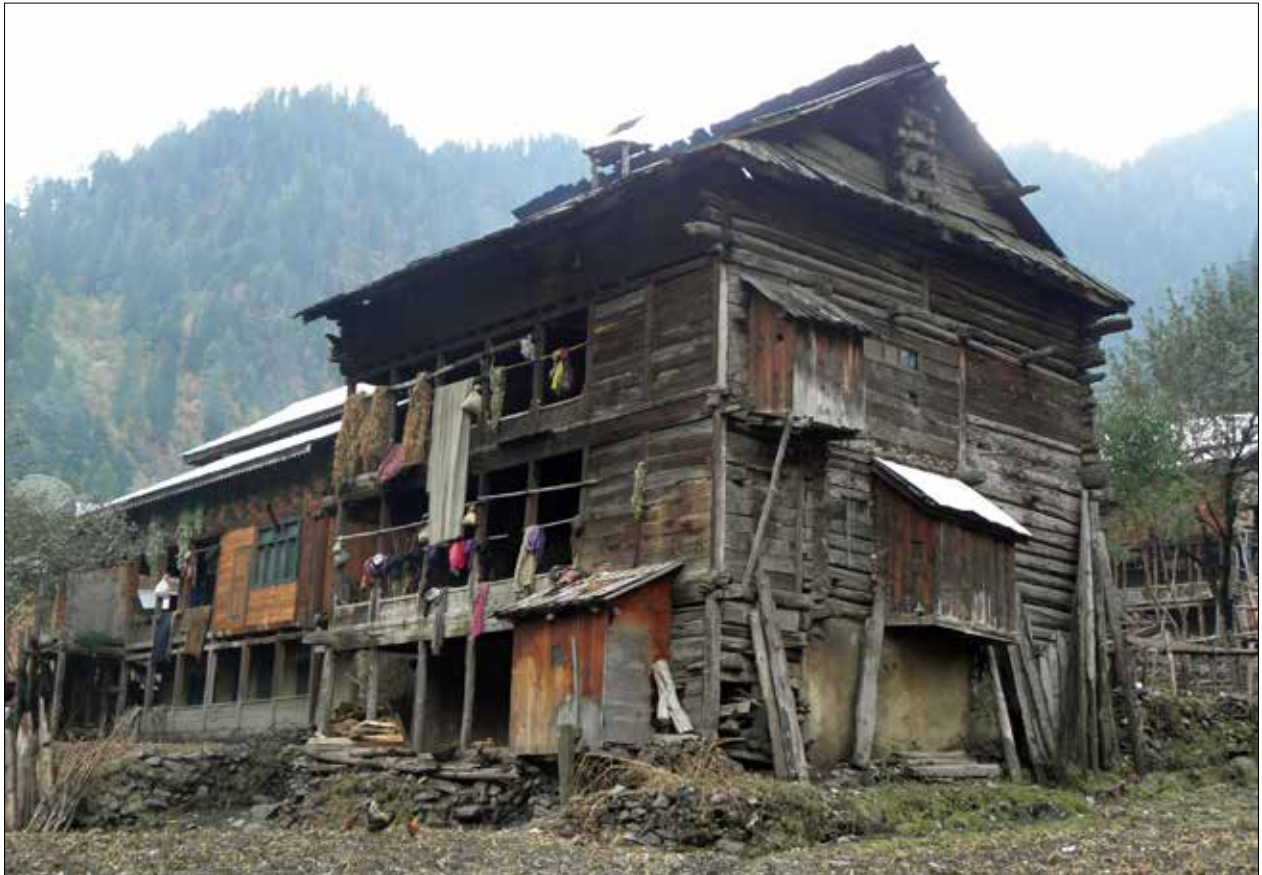
Figure 11. Projecting washrooms in three floors, based on cantilever principle (Photograph: Authors).
