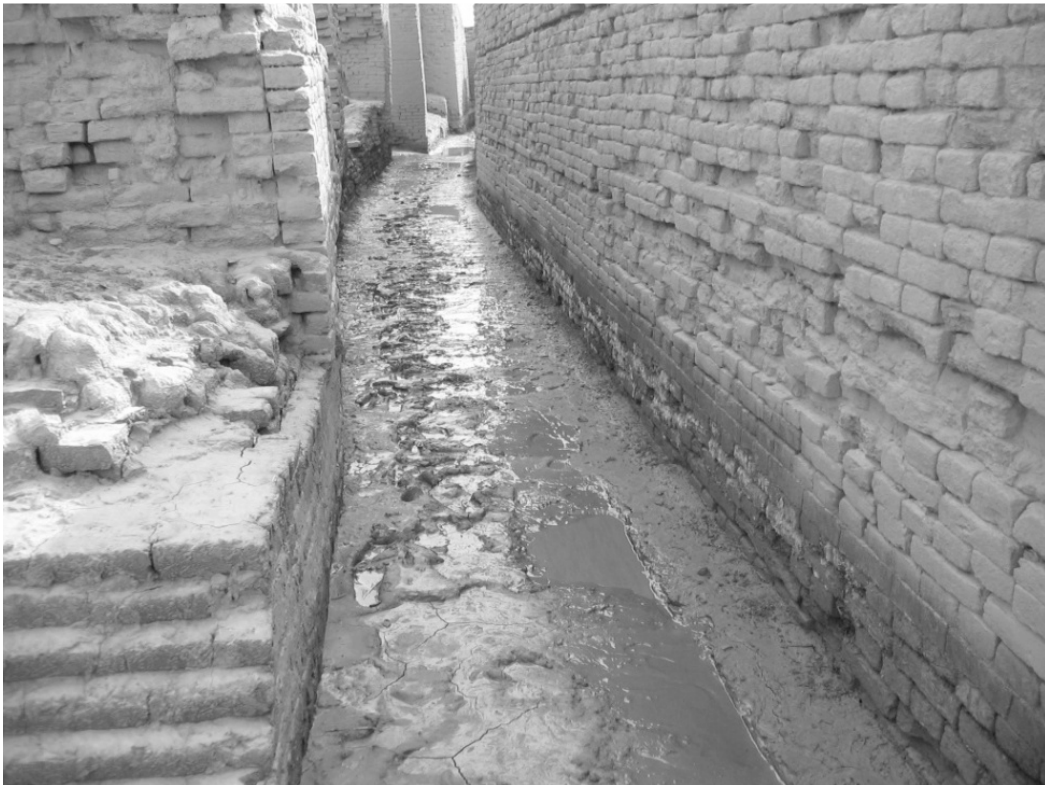
Figure 5: Moenjodaro, Water ponding after monsoon rain, DK-G area.
