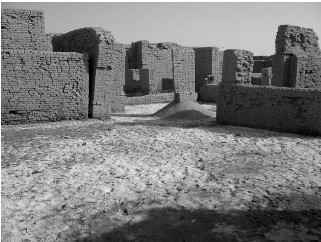
Figure 4: Moenjodaro, Picture showing DK-G area with salts affected soil.
