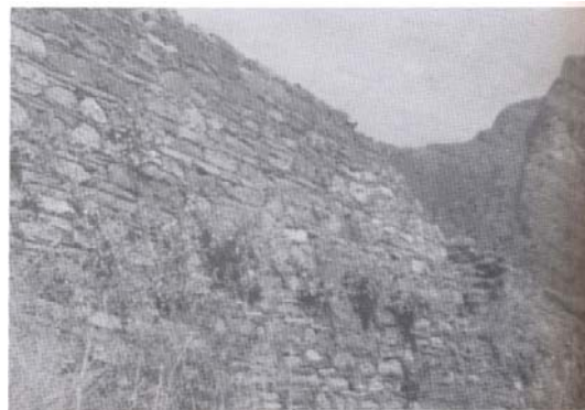
Pl. 3. Chancher. A huge retaining wall constructed of stone secured from ancient monuments.
