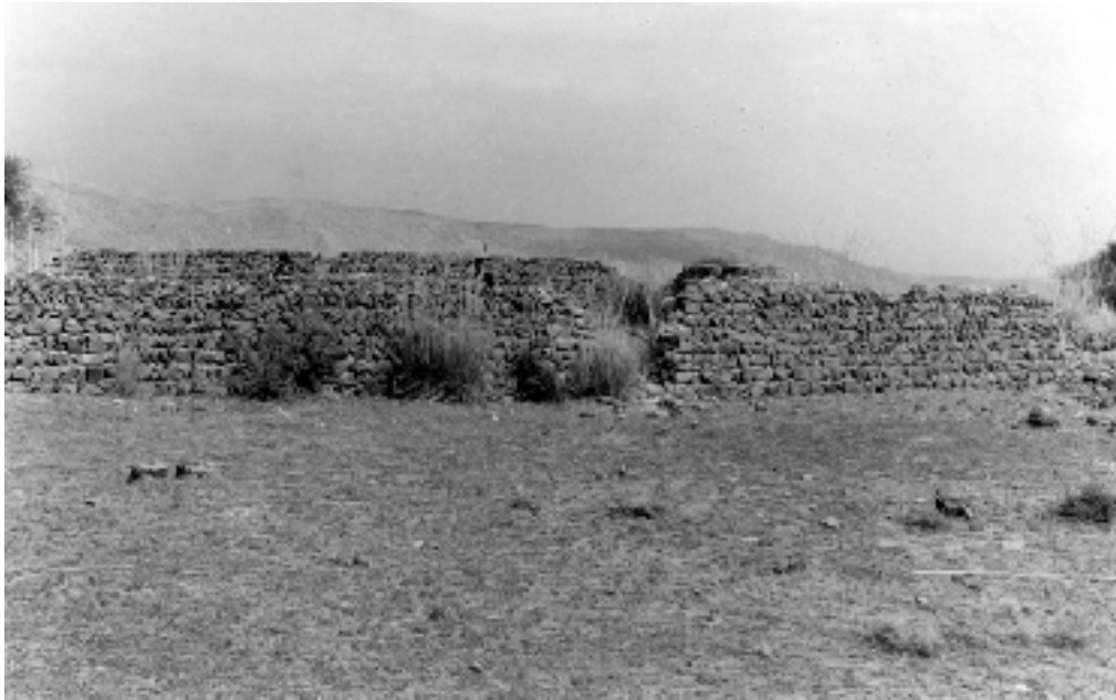
Pl. 3a. Karak (Sultan Sh āh Nika): A long wall in residential area built of local stones and lime mortar.
