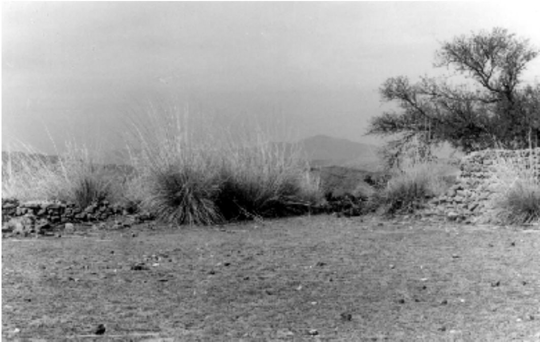
Pl. 2a. Karak (Sultan Shāh Nika): Residential area with broken walls and wild shrubs.
