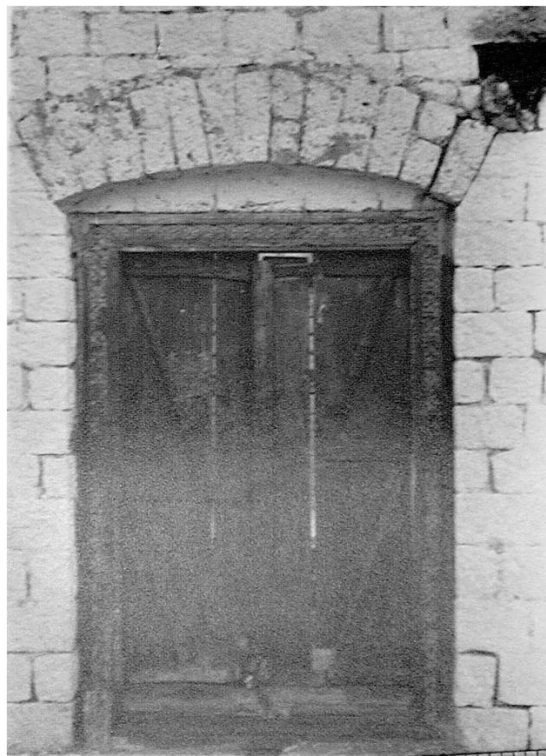
Pl. 3: Kohat (Karbogha): Entrance to the Tomb building under a segmental arch and wooden door.
