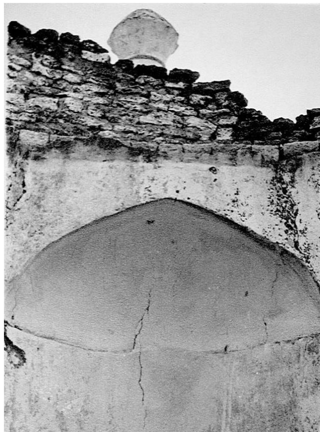
Pl. 5. Kohat (Karbogha): Phase of transition showing the squinch Arch, projected corners and missing dome
