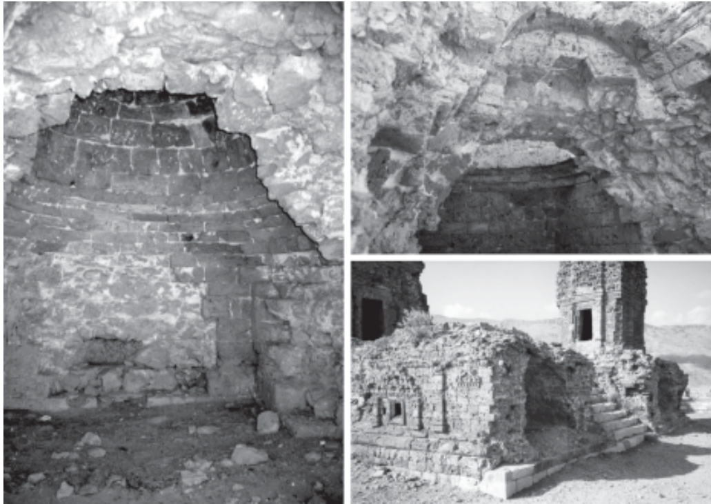
Pl. 7: Bilot Kafirkot, Temple D, southeast chamber in platform extension. Temple E subshrine is visible to the northeast.
