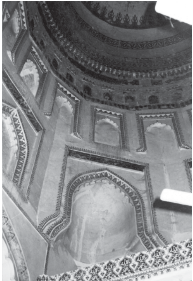
Plate IV: Tomb of Pir Adil in District Dera Ghazi Khan showing zone of transition
