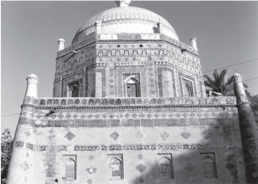
Plate III: Tomb of Pir Adil in District Dera Ghazi Khan showing second and third storey from west side
