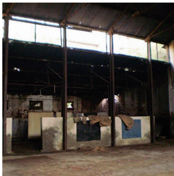
Figure 9. Steel Section (I-Columns) (Photograph: Author)
