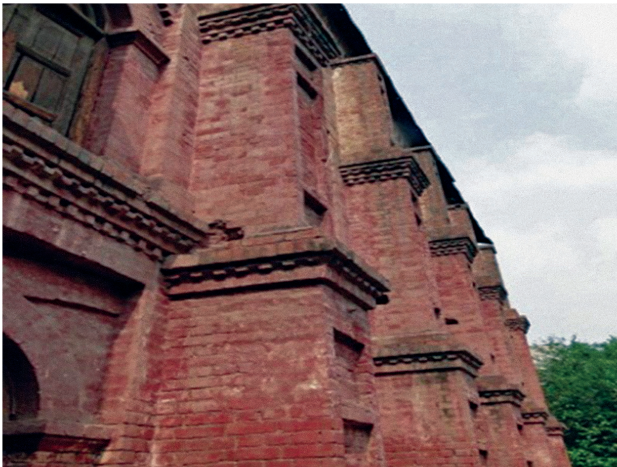
Figure 7. Buttresses on the external façade (Photograph: Author)
