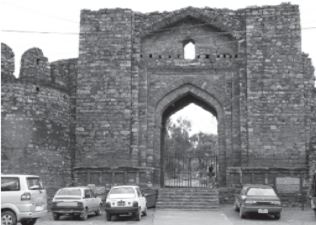
Pl. I. Rawat: General View of the Eastern Gateway
