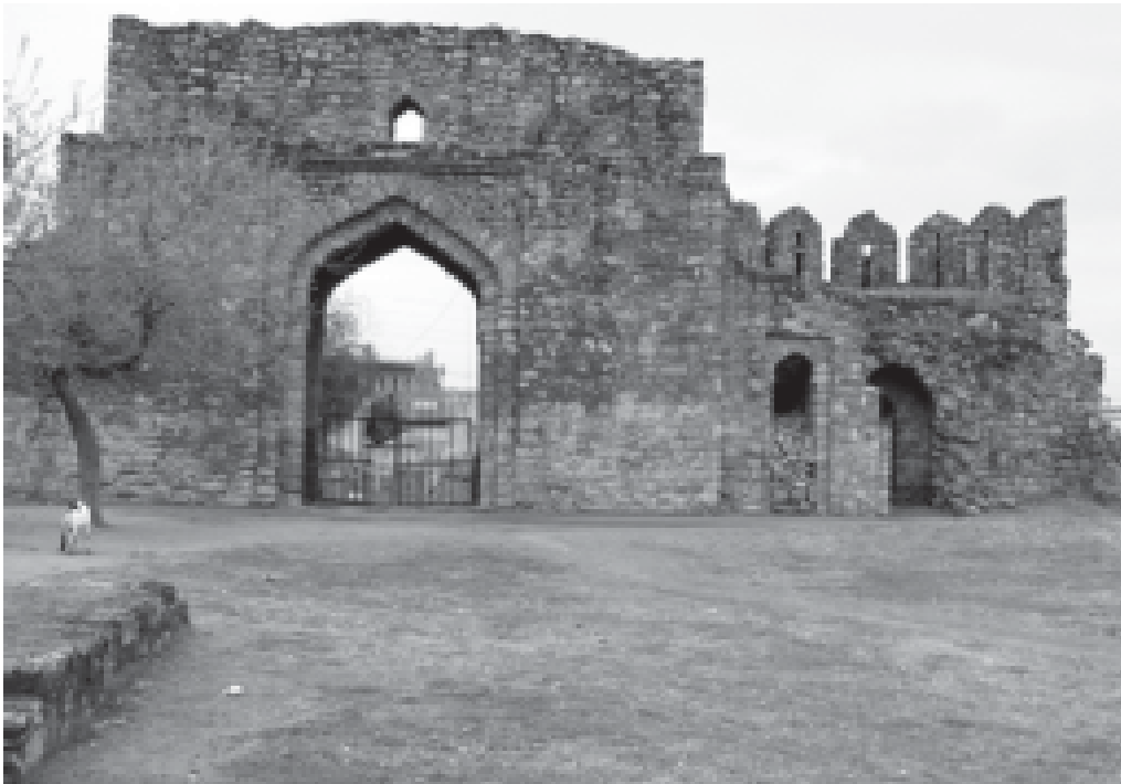
Pl.II Rawat : A View of the Eastern Gateway from the inner courtyard
