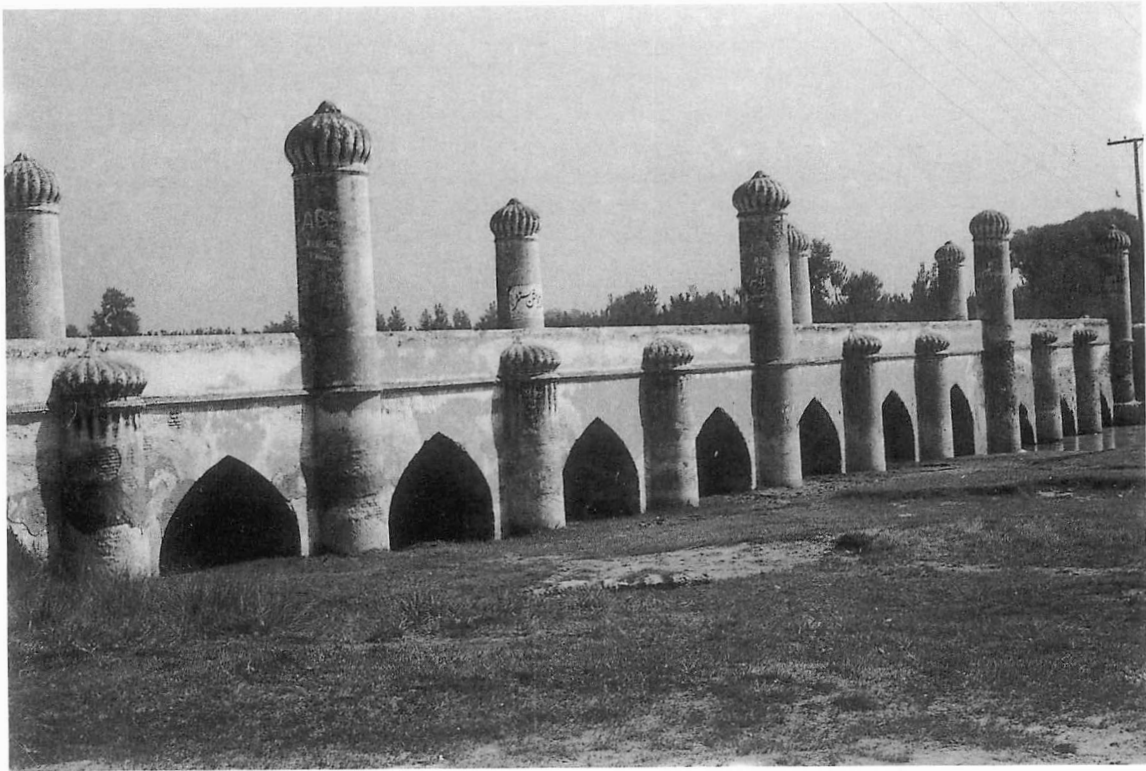
Pl. 1: Chamkani: Chu'a Gujar Bridge on the Bārā stream.
