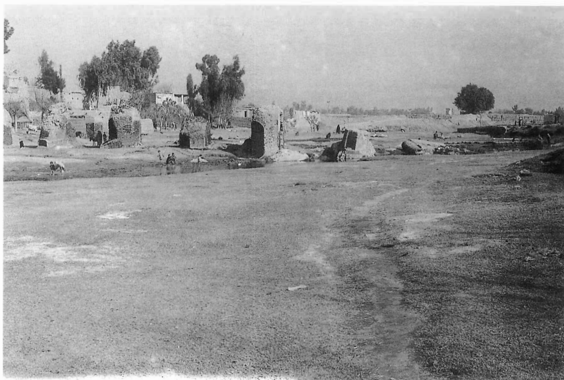
Pl. 3: Zinda'i Bridge: View from the south.
