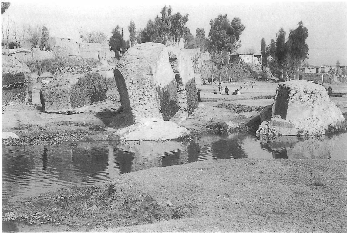
Pl. 9: Zinda'i Bridge: View of the piers from south side showing sharp pointed ends.
