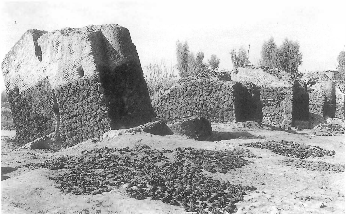
Pl. 7: Zinda'i Bridge: Surviving remains of the bridge.
