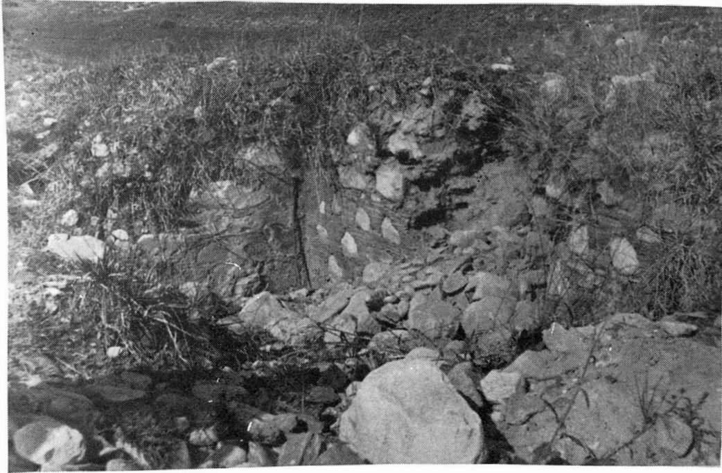
a. Rashaka: Structure of diaper masonry.
