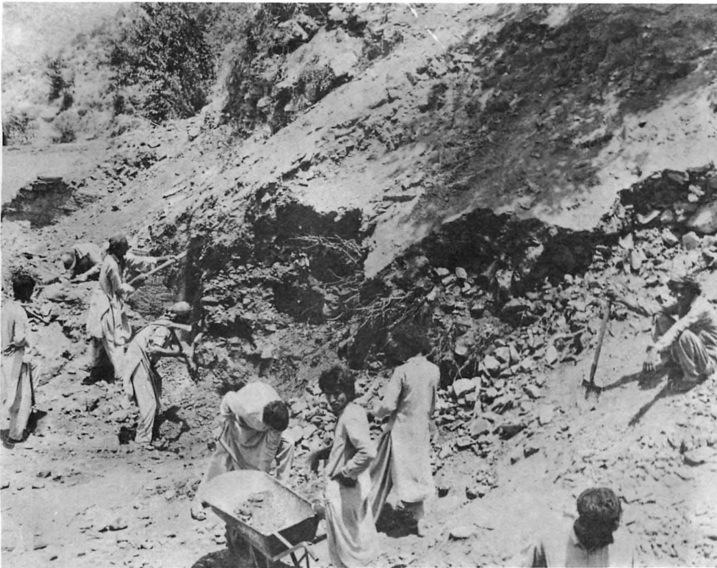
Pl. IIIa. Shnaisha: Removing the pile of debris from the west side.
