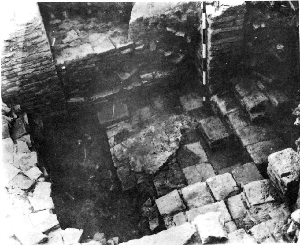
Pl. IIIa. Manṣūra: View from N.N.W. Two periods of brick paved floor in Sq. No. ASXXX/21.
