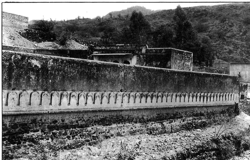
Pl. 10. Attock: Bahram-ki-Baradari General view showing the western perimeter wall with merloned band in the middle.
