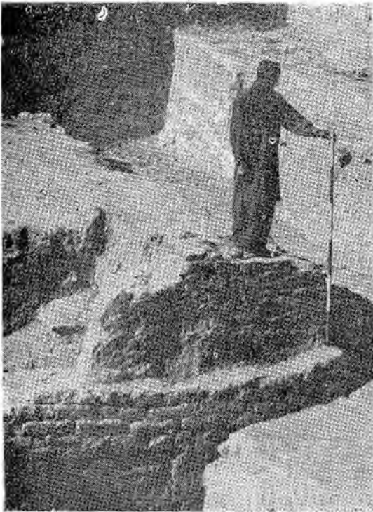
No. 3. A11'—Corner wall in the main street
