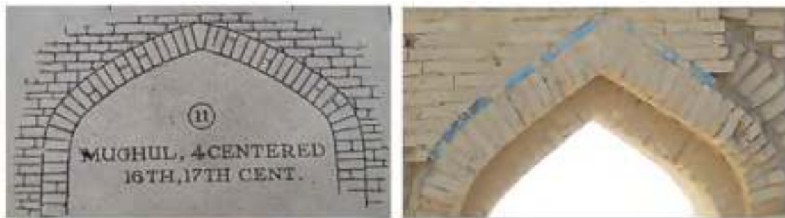
Plate 19. On the left showing Mughal Period arch and on the right an arch of the Sooran Tomb (Courtesy Percy Brown).
