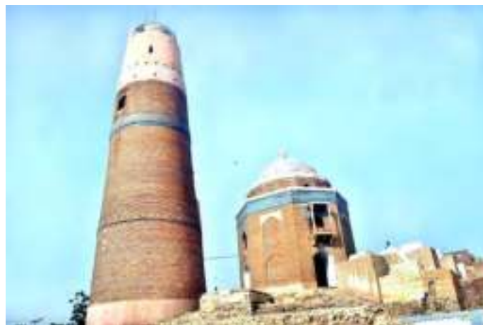
Plate 23. The tomb of Meer Masoom Bakari with the tall tower in Sukur (courtesy google)
