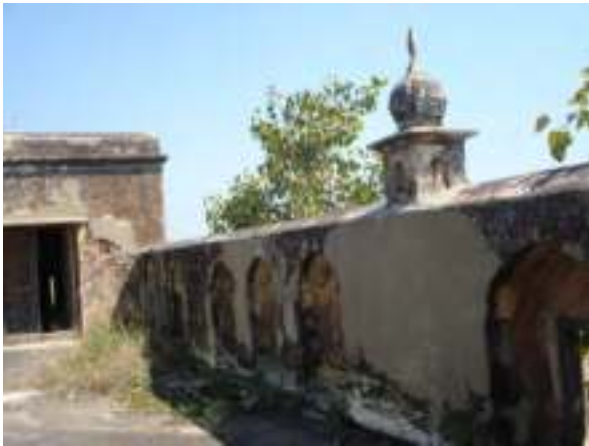
Plate 21: Viwe of the guardroom and parapet wall
