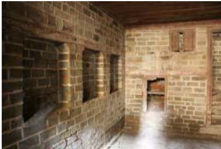
Plate 23: View of the basement
