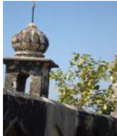
Plate 22: close up view of the kiosk
