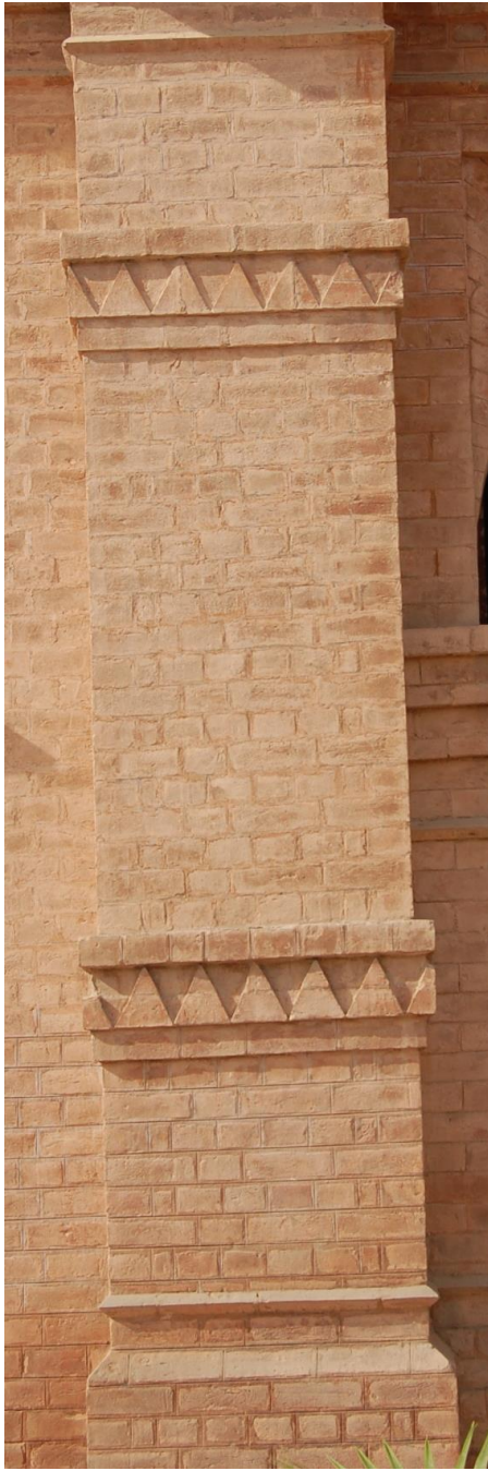
(Plate 13 Square Shaped Column)
