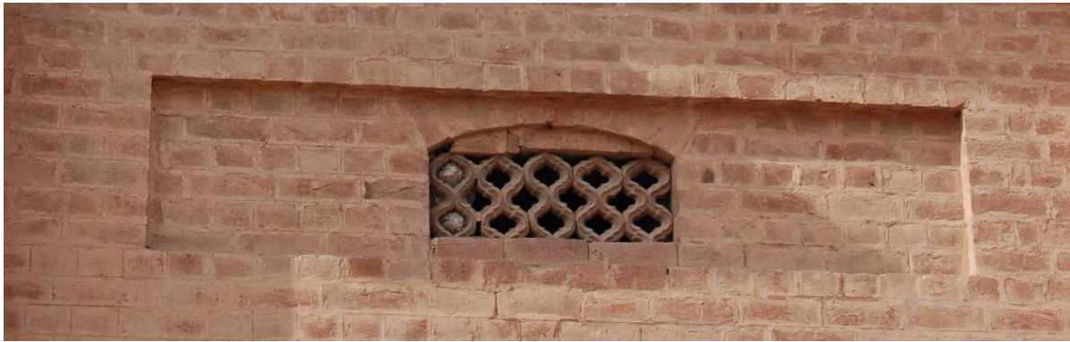
(Plate 11 Fret Work Ventilator)
