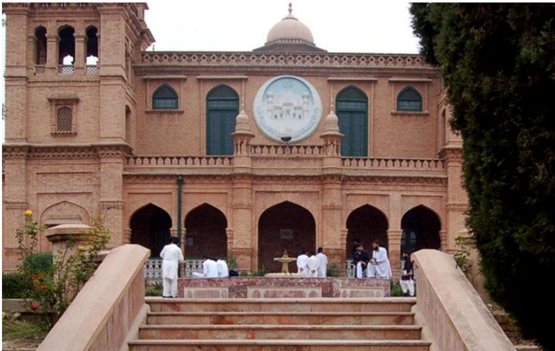
(Plate 2: Back Façade of College)
