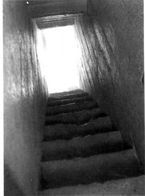
Fig. 4. Tomb of the sister of Jam Fateh Khan: stairs leading to the roof
