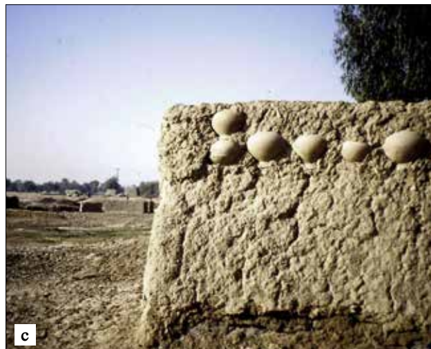
Figure 10. (a) A communal horseshoe shaped sloping kiln (9.5 m long by 2.8 m wide, height ranging from 0.6 to 1.5 m) located in an open space in the village of Gandhi Khan Khel. (b), (c) 'Wasters' are not wasted: misfired reject pots are put to use in wall construction (village Gandhi Khan Khel).
