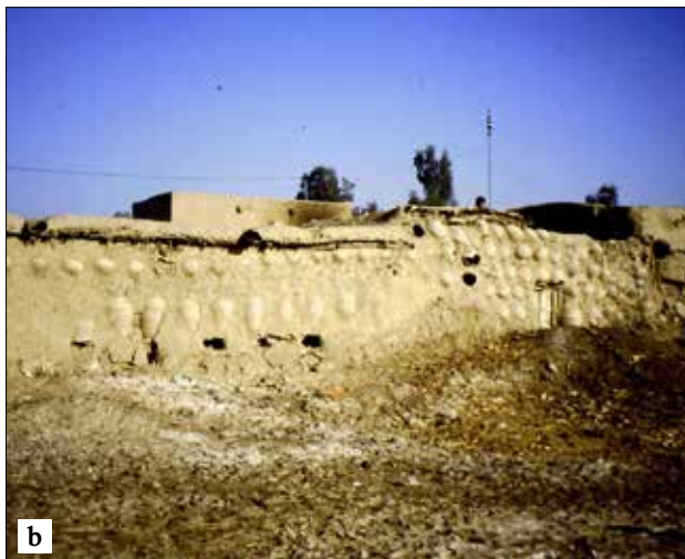
Figure 10. (a) A communal horseshoe shaped sloping kiln (9.5 m long by 2.8 m wide, height ranging from 0.6 to 1.5 m) located in an open space in the village of Gandhi Khan Khel. (b), (c) 'Wasters' are not wasted: misfired reject pots are put to use in wall construction (village Gandhi Khan Khel).
