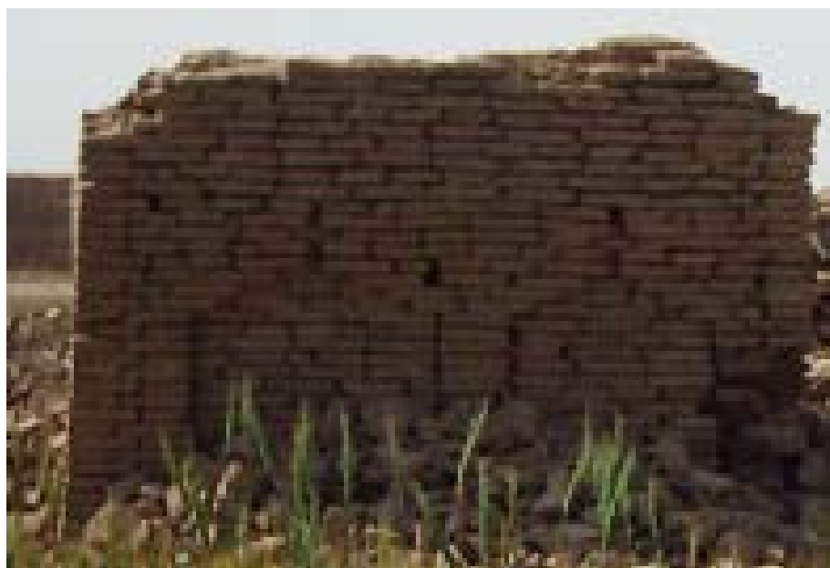
B. Eastern wall showing details of sunk Arches
