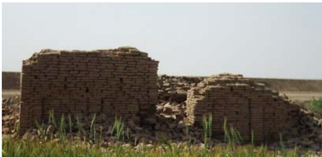
A. General view of the structure
