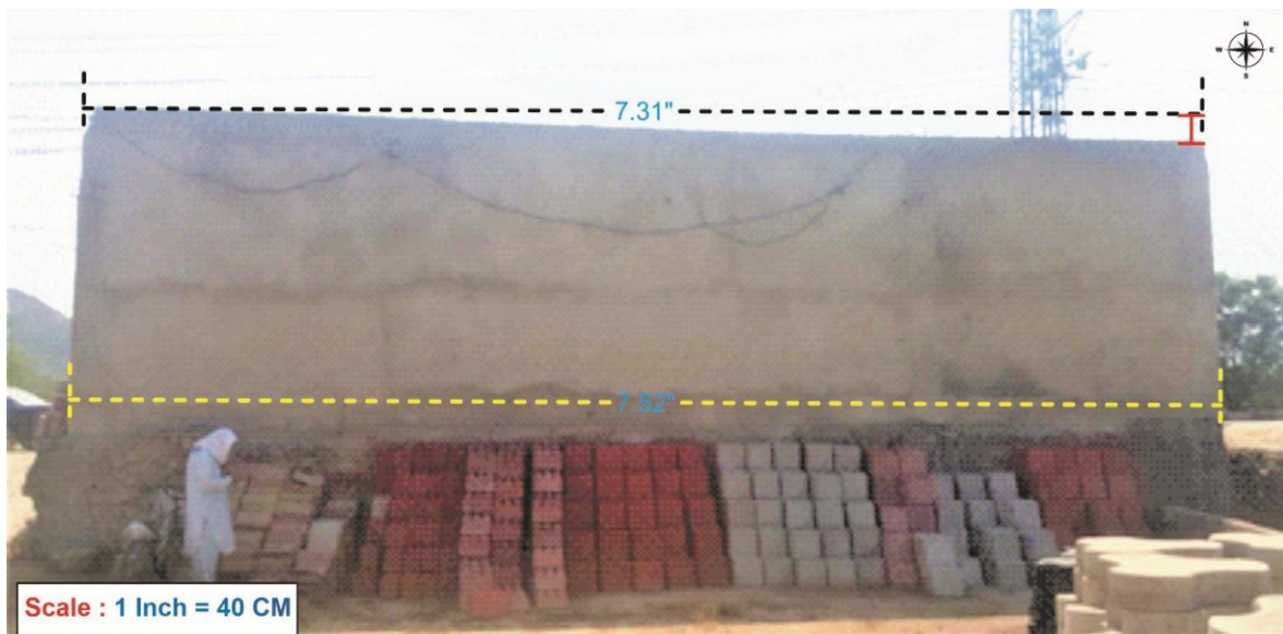
Fig. 7. A photograph was taken at a 90° angle showing a 7cm subsidence on the eastern side of the building.
