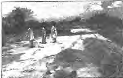
Photo 18. A view of a village (Tobo) southwest of Diplo located at the crest of a stable dune. Some 20-30 mud and cane houses completely or partially collapsed in response to fractures related with the lateral spreading.
