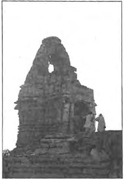
Photo 6. An historical Hindu temple near Nagar Parkar suffering partial collapse in response to ground shaking.
