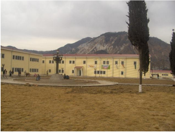
Fig. 3. Main University Building, CMH Road, Muzaffarabad (2-story steel frame structure constructed after the earthquake).
