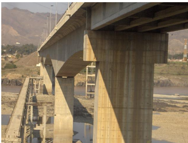
Fig. 5. Continuous RC box girder, New Khairabad Bridge, on River Indus GT Road (N5).
