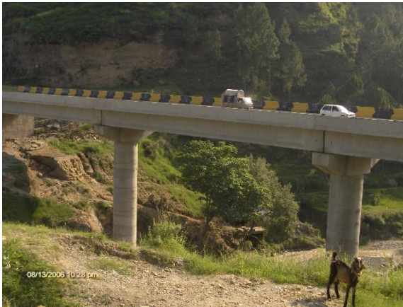
Fig. 4. Three-span RC Bridge near Mansehra (Mansehra-Balakot Road).
