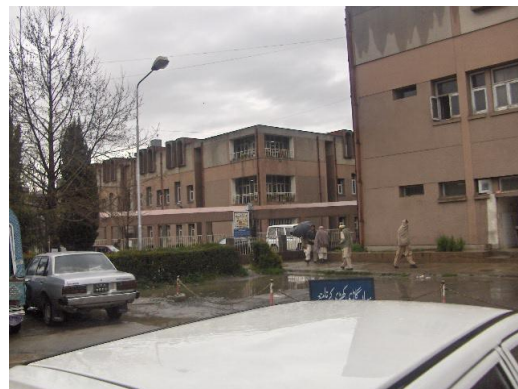
Fig. 2. Ayub Medical Complex (AMC) Hospital Abbottabad (3-story RC frame structure).
