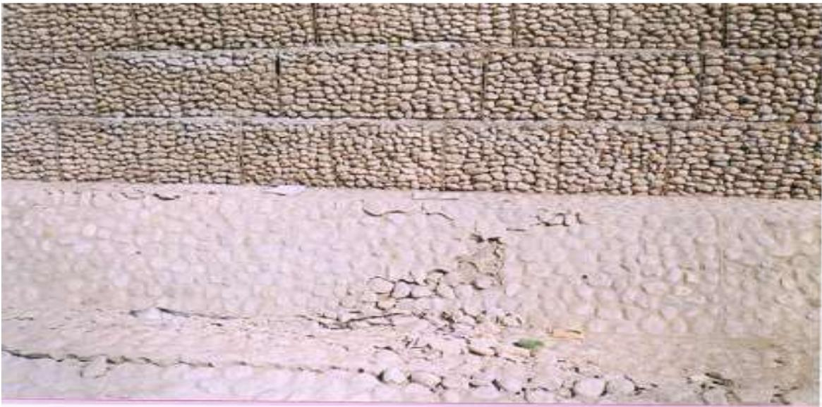
Fig. 1. B: heaving effect in the retaining wall at the toe of the slope.
