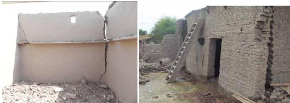
Fig. 5. Damaged houses due to splitting of corners.
