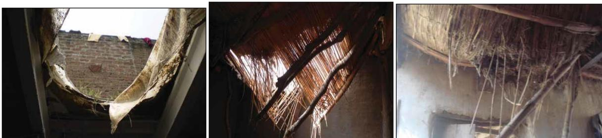
Fig. 6. Damaged roofs of the mud houses.
