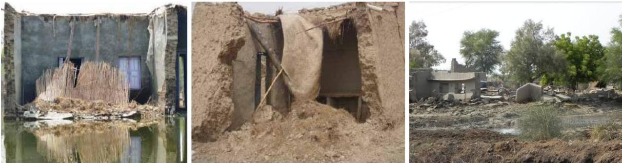
Fig. 7. Flood damaged houses due to wiping out of houses mostly located in the flood plains.
