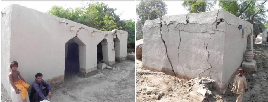
Fig. 4. The damaged houses due to undermining of the foundation by flood water.
