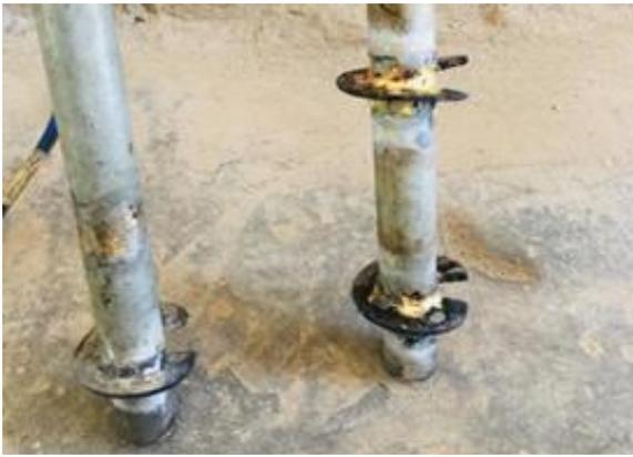
Fig. 6. Single Helix and Double Helix pile.
