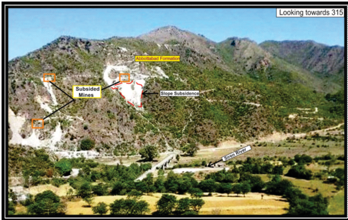
Fig. 1. Shows the large-scale mine subsidence in village Bheer, Haripur Hazara (Figure Not according to Scale)
