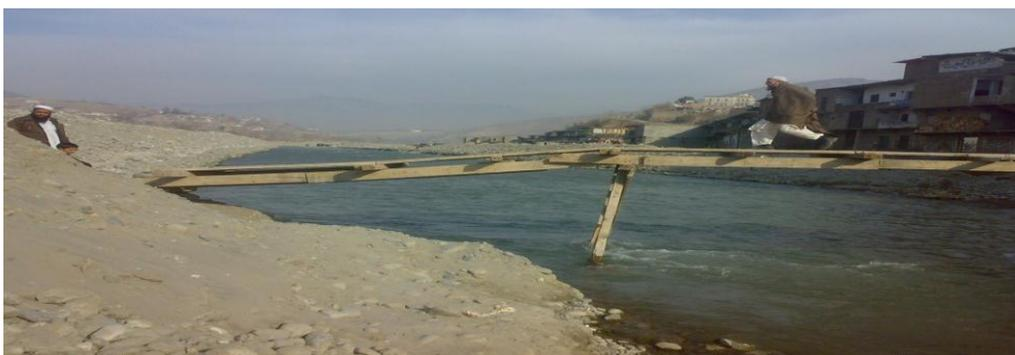
**Fig. 8: Temporary wooden bridges constructed by the community**
